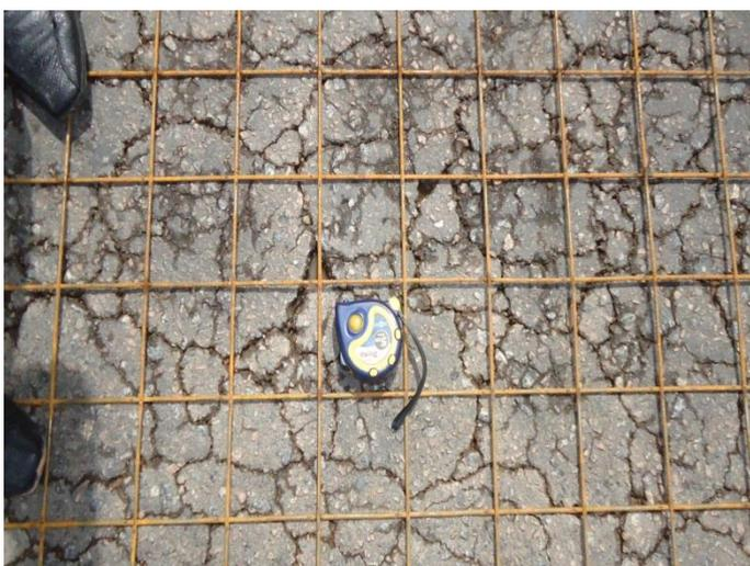
Figure 6. “Crocodile cracks” on existing pavement.
