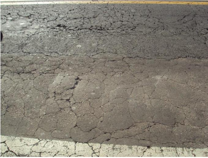
Figure 1. SP354 view of the pavement in the presence of 100% defect "crocodile crack".
