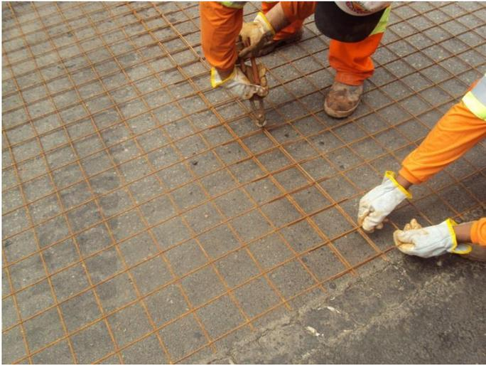
Figure 5. Fixation of the steel mesh.
