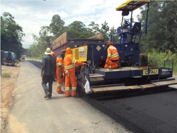
Figure 3. Repaving applied using asphaltic concrete.
