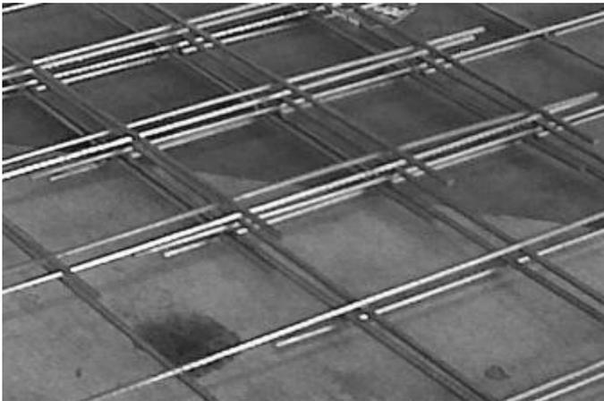
Figure 2. Detail of overlapping meshes.
