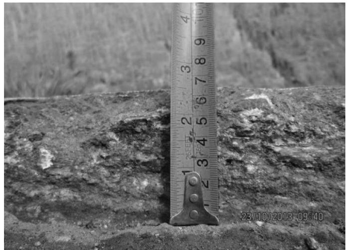
Figure 4. 6 cm of thickness milling.
