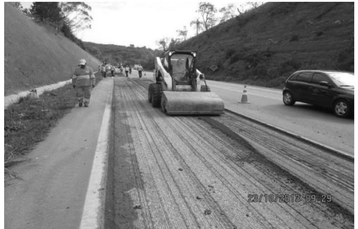
Figure 3. Pavement milling.
